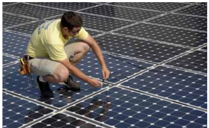
Illustration 8. Man wiring solar panels
